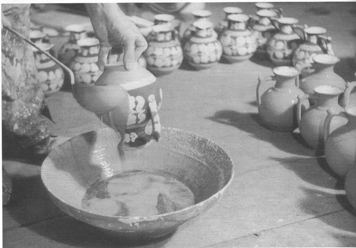
26 Polievanie džbánov glazúrou, Pozdišovce 1955 Glazing a pitcher, Pozdišovce 1955
